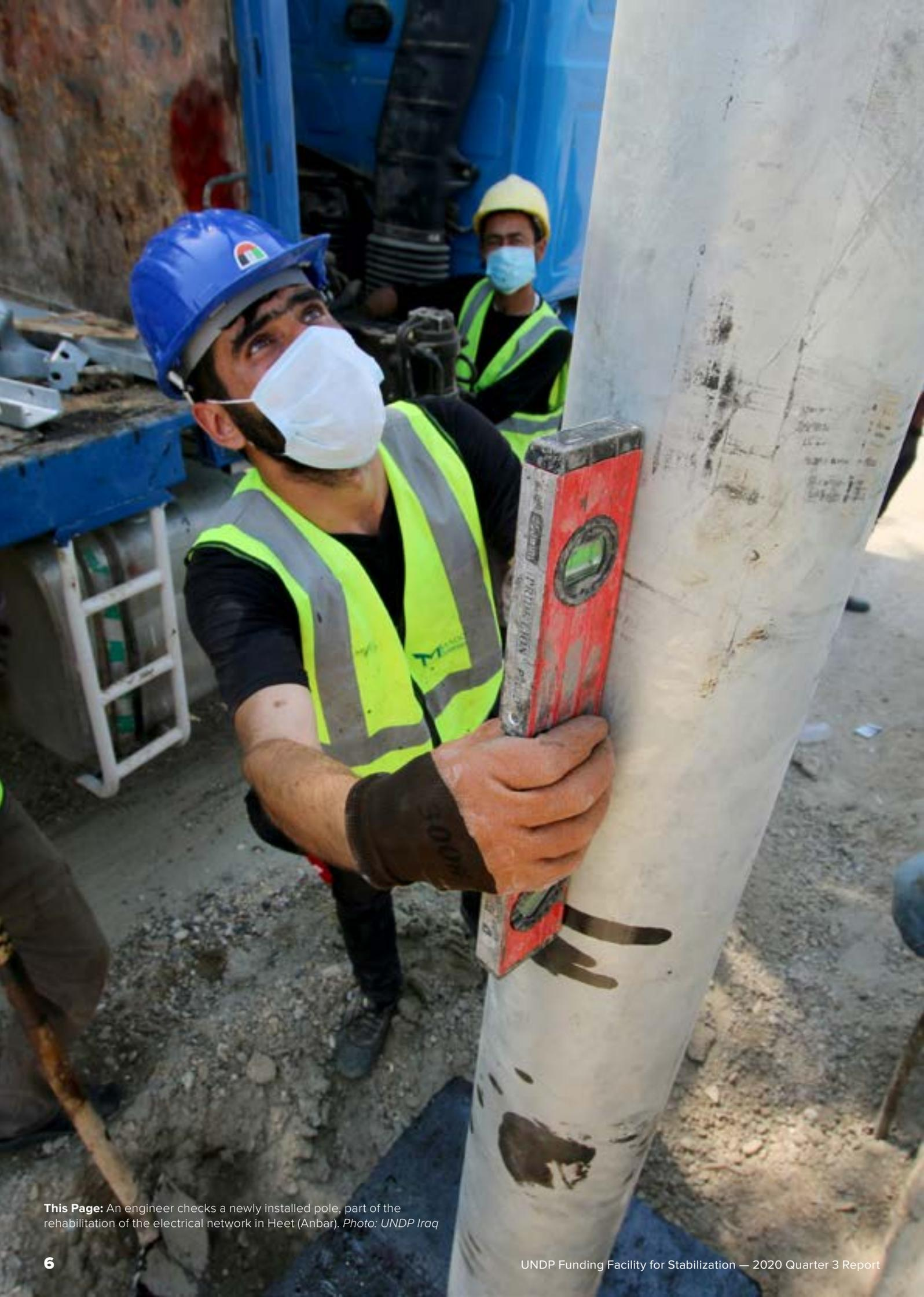
**This Page:** An engineer checks a newly installed pole, part of the rehabilitation of the electrical network in Heet (Anbar). *Photo: UNDP Iraq*
